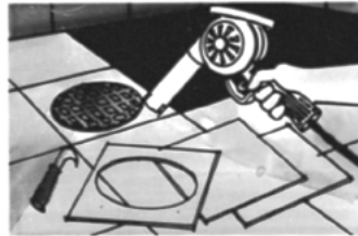
SOFTEN FLOOR TILE
